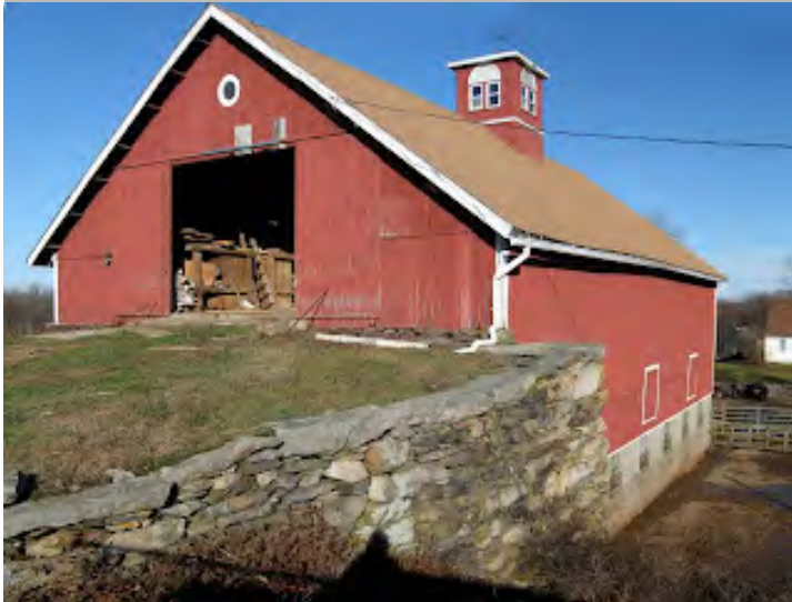
Hay Barn with Ramp to Unload the Hay Wagon into the High Drive
